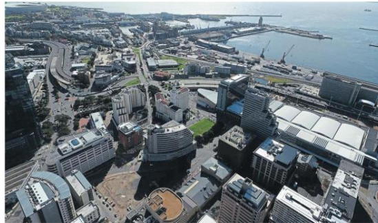
The unfinished bridges in the Foreshore. PHOTO: SUPPLIED
