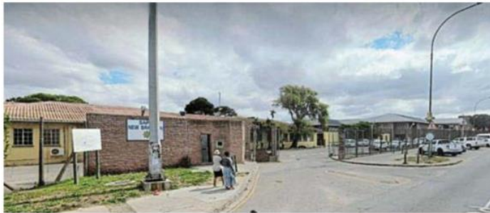
CRUMBLING AWAY: The New Brighton police station is in extremely poor condition, according to an auditor-general report Photograph: GOOGLE MAPS
