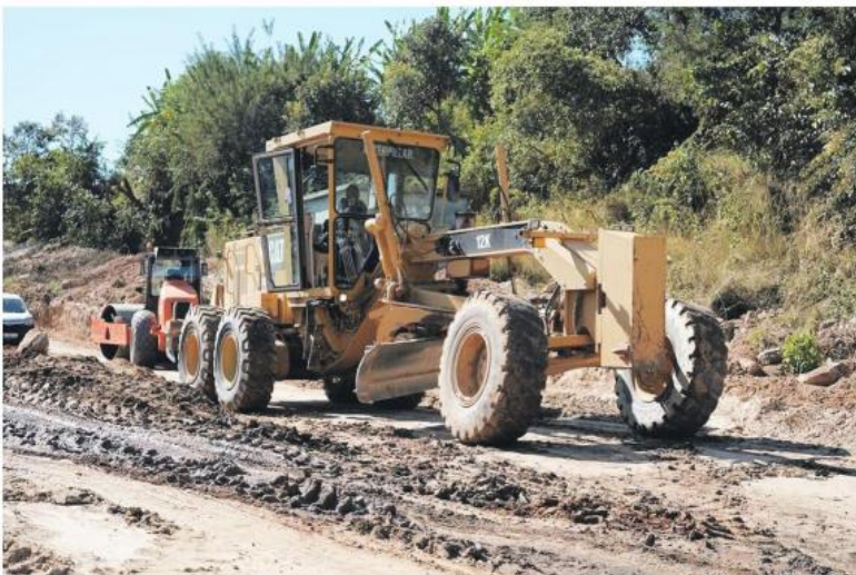
The D3179 road is being rehabilitated.
