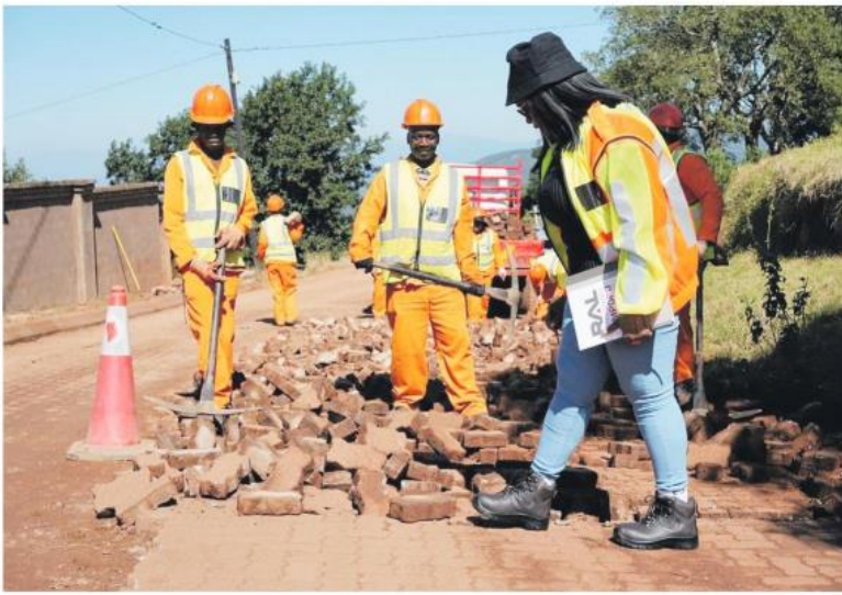
RAL repairs pavements.
