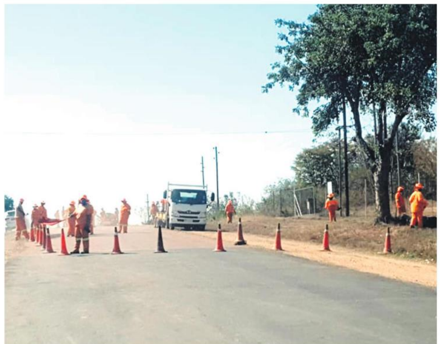
Eiland road construction in progress. > Photo: Supplied
