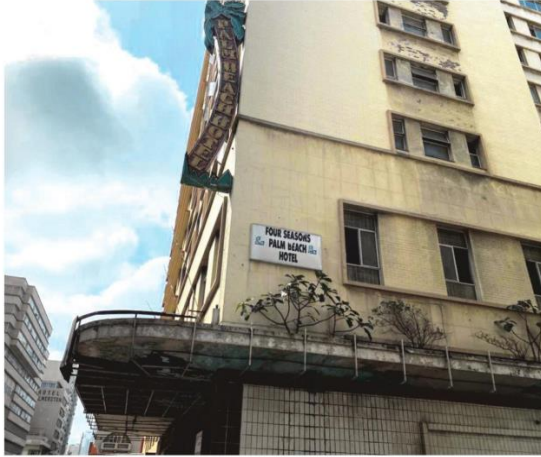
The abandoned Palm Beach Hotel in south beach Durban is one of 14 properties that eThekweni Municipality is looking into converting into accommodation for the April flood victims. PHOTO: THABISO GOBA
