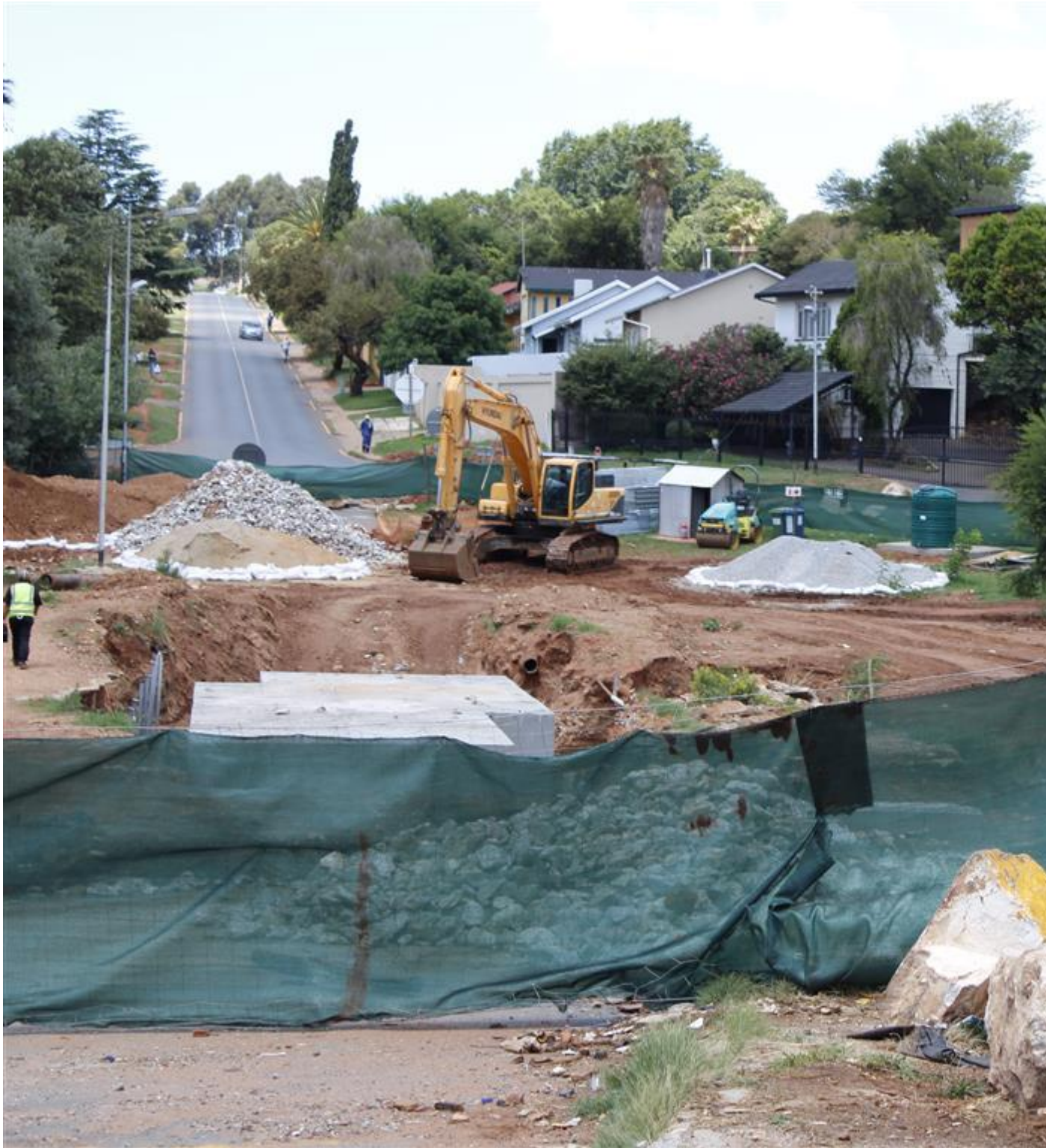
The closed bridge on South Road. Photo credit Amy Slocombe
