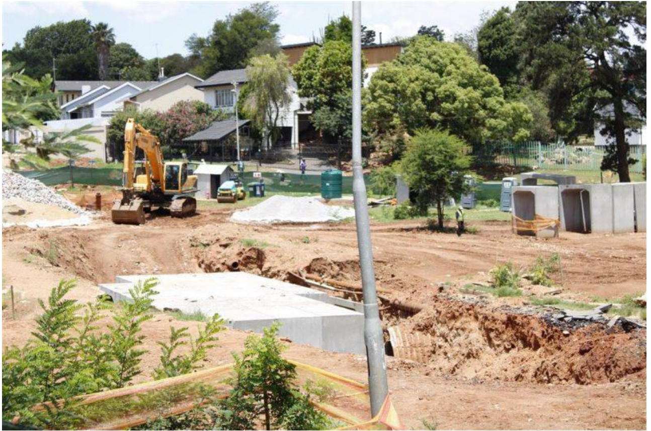
The closed bridge on South Road. Photo credit Amy Slocombe
