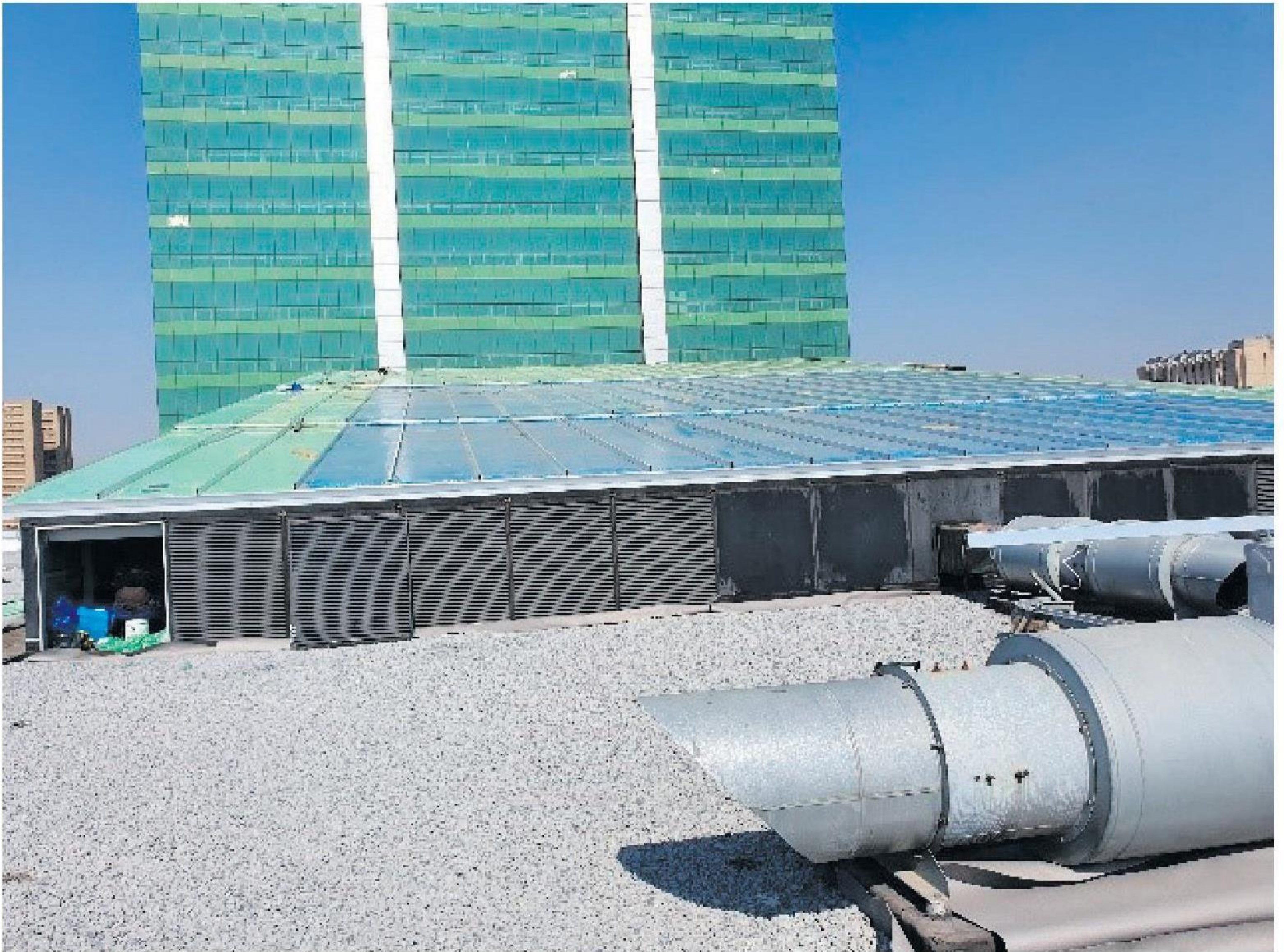
Roof and chillers being renovated at Civitas.
