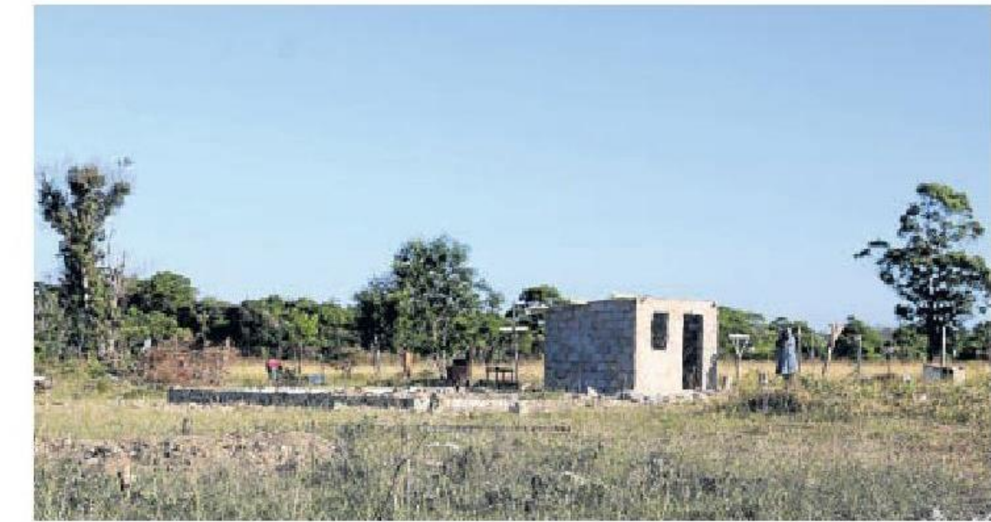
DESERTED; The shell of a demolished house at Farm 924 on Friday.
