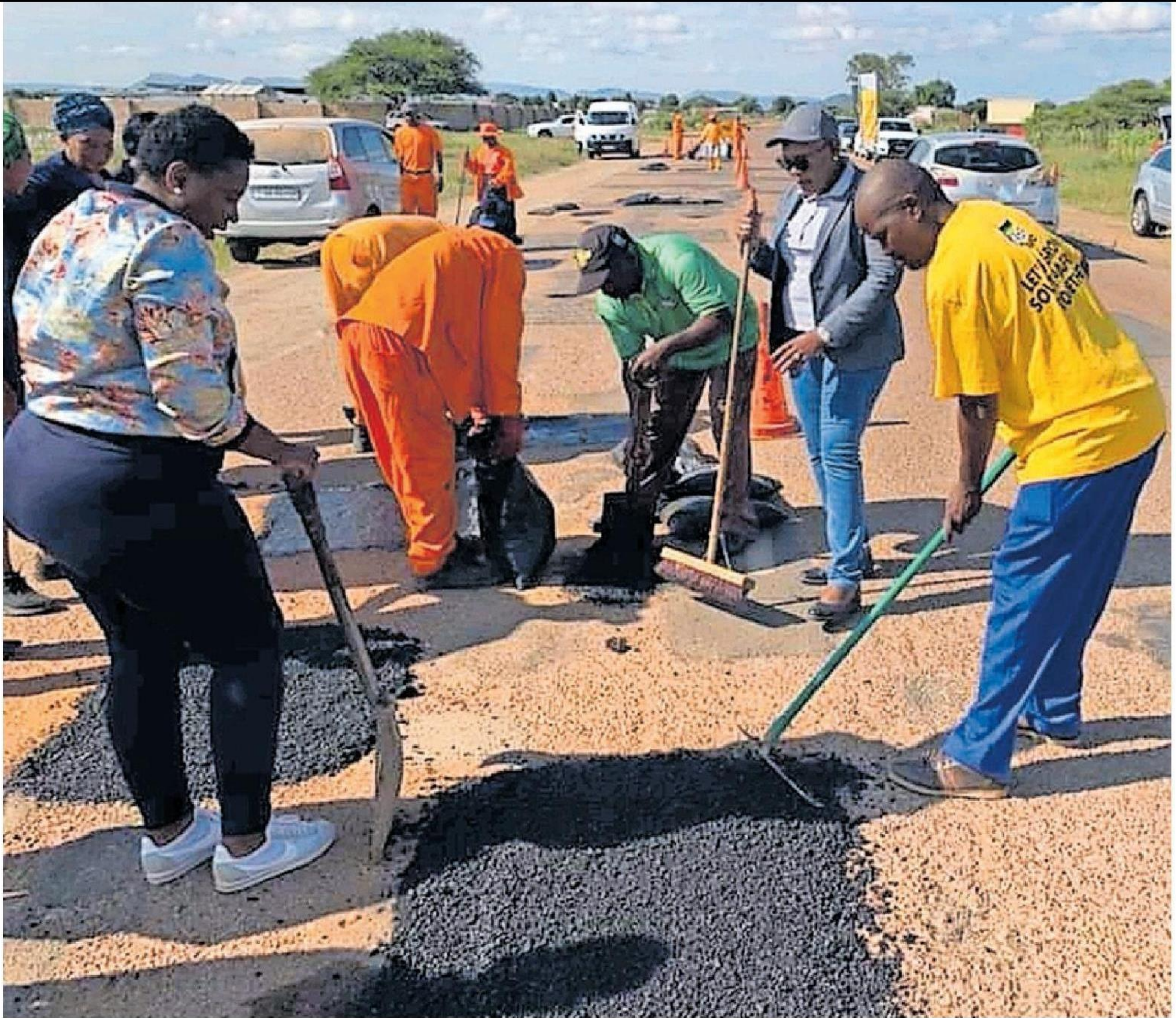
Public Works MEC Nandi Ndalane, assists workers in fixing a pothole.
