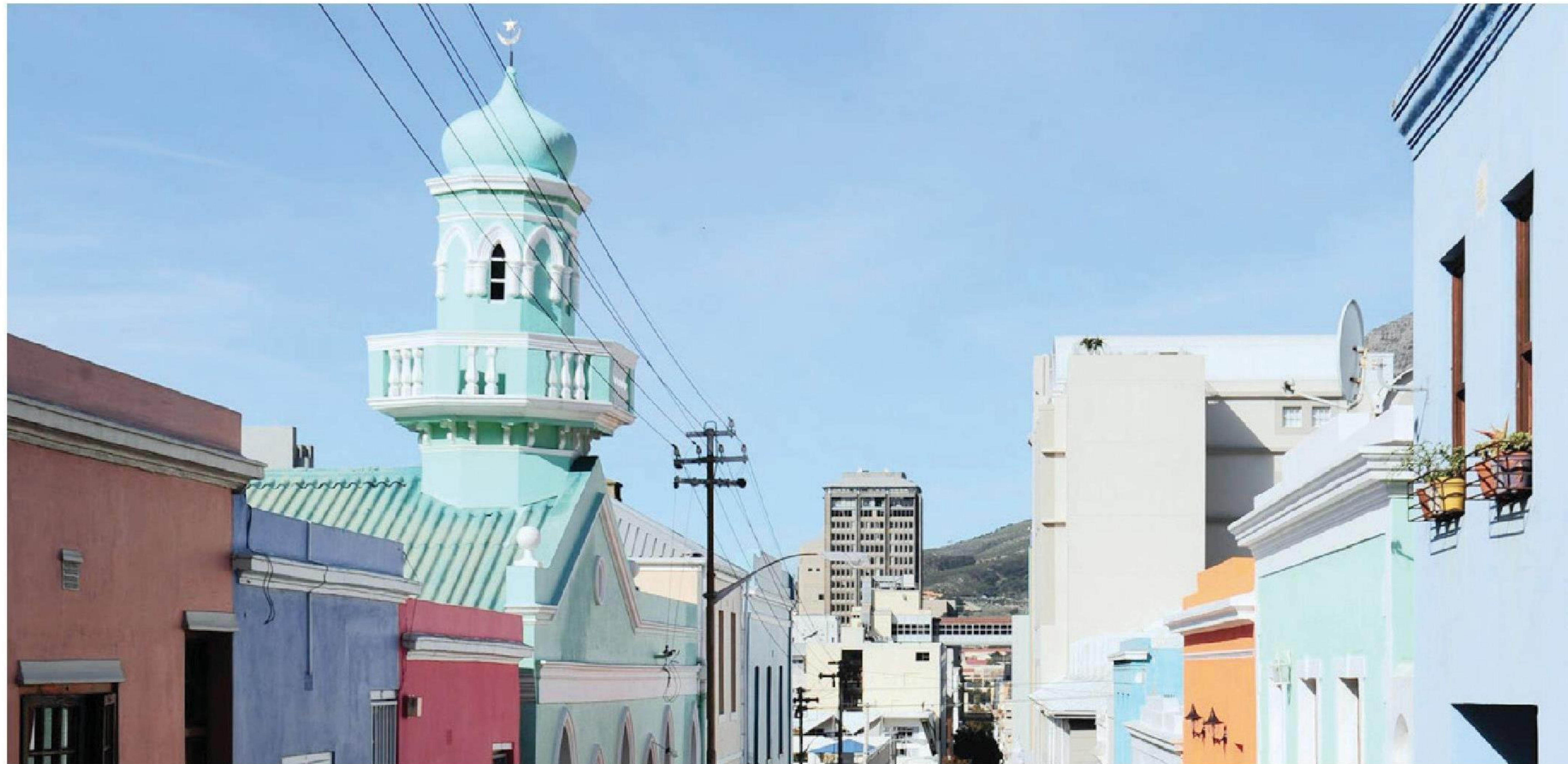
THE Boorhaanol mosque is one of 19 sites in Bo-Kaap declared Heritage Sites. | HENK KRUGER African News Agency (ANA)
