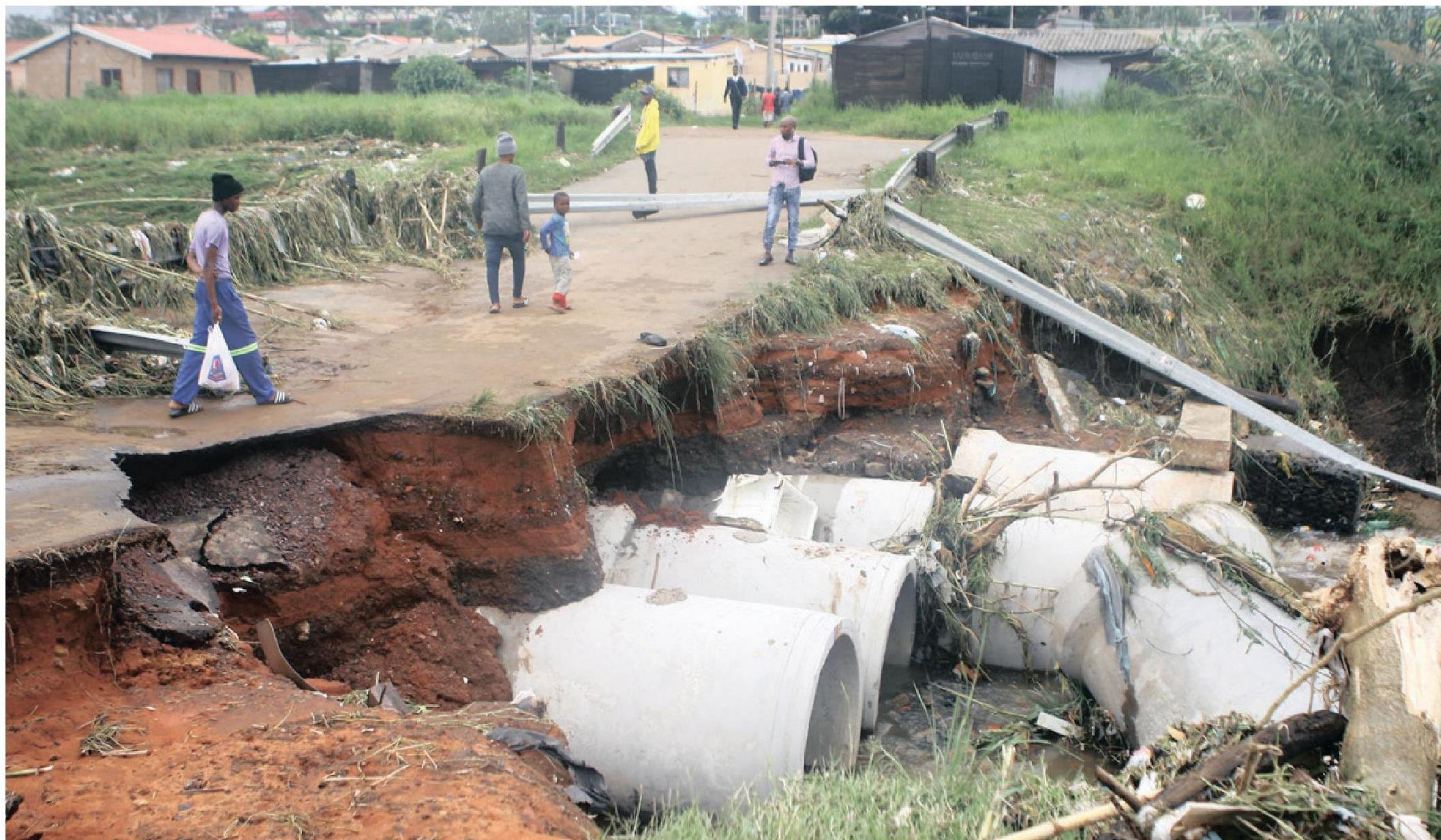
A temporary bridge that collapsed after a stream flooded during a thunderstorm on Sunday afternoon.
