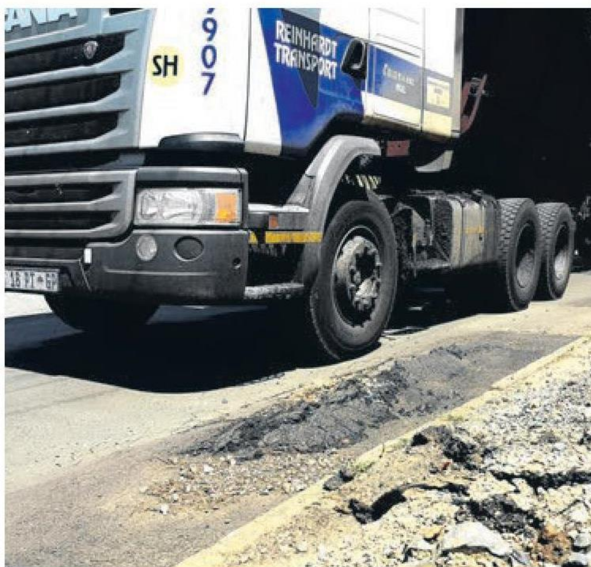
The new repairs are only two weeks old and have again started to lift and crack
