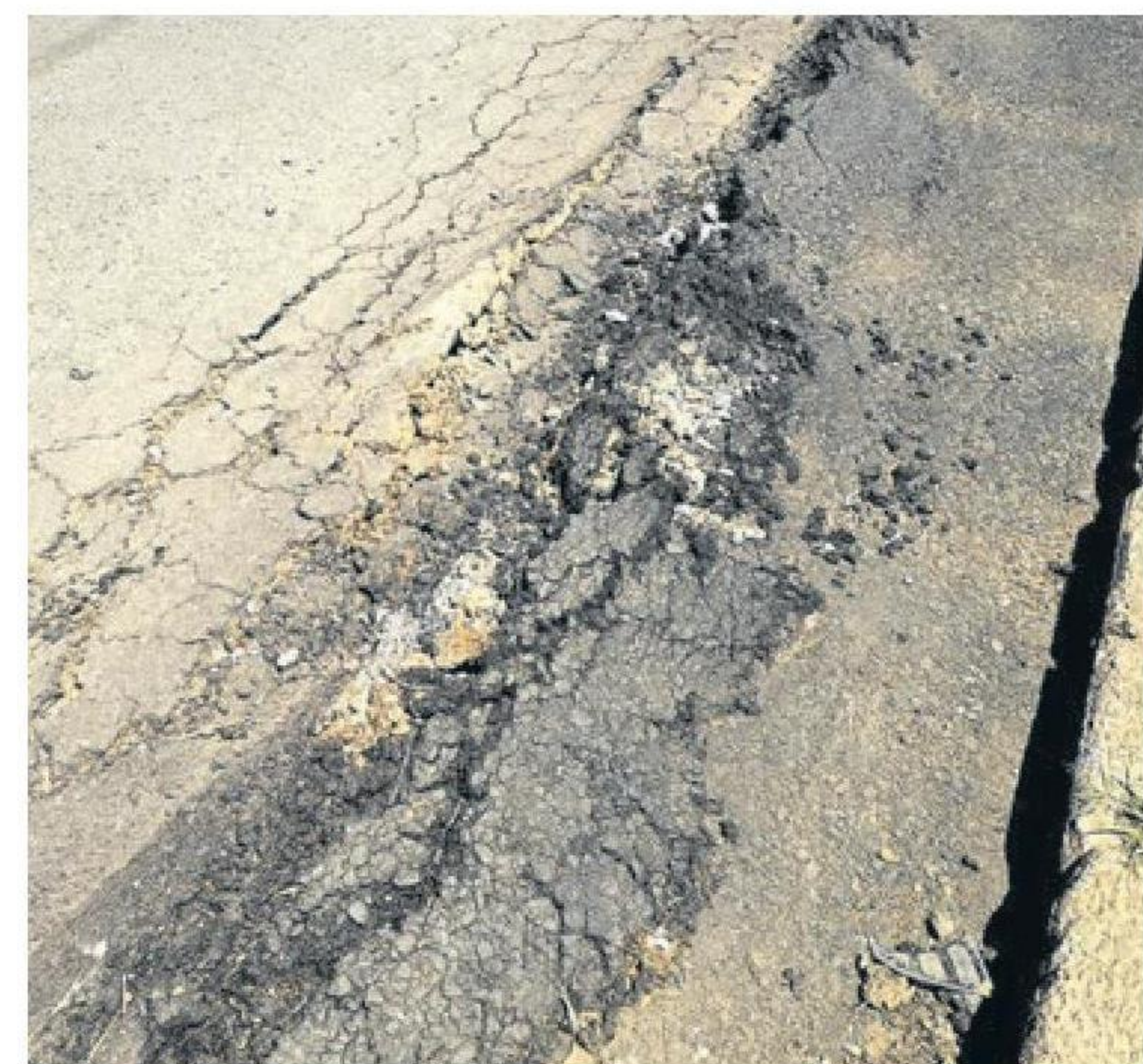
The new repairs are only two weeks old and have again started to lift and crack
