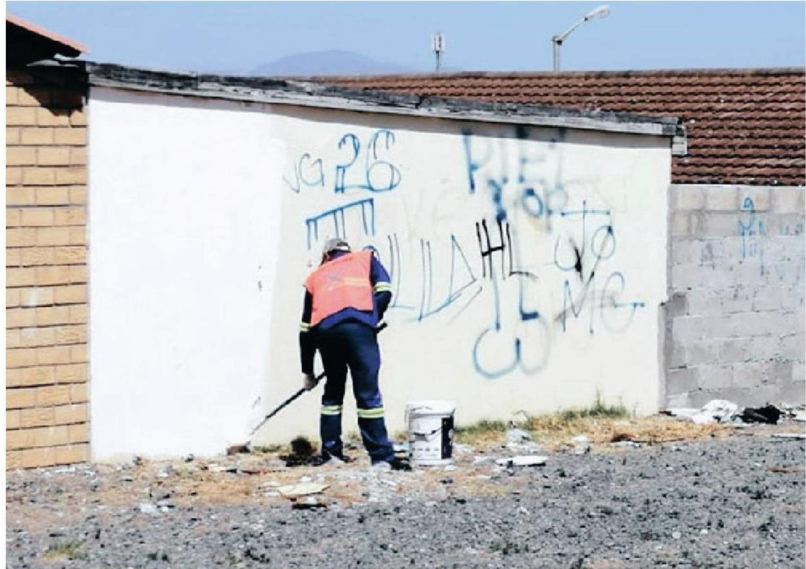
■ An EPWP worker removes graffiti from a wall in Woodlands.
