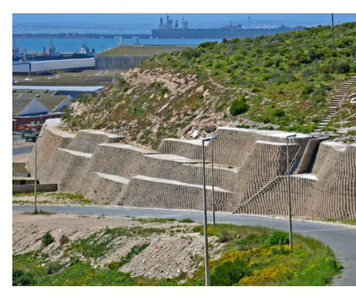
A large-scale erosion-control retaining wall to stabilise the existing eroded embankments in the Pepper Bay harbour area on the West Coast was initiated in the interest of public safety by the Department of Public Works.
