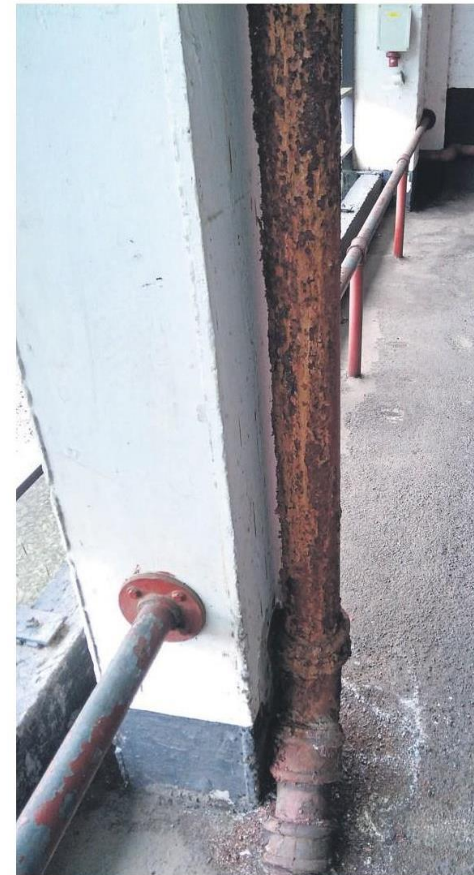
ABOVE: A rusted water pipe at the Davis Alexander Building. LEFT: Garbage piles up in a disused toilet cubicle in the Davis Alexander Building. PHOTOS: KERUSHUN PILLAY
