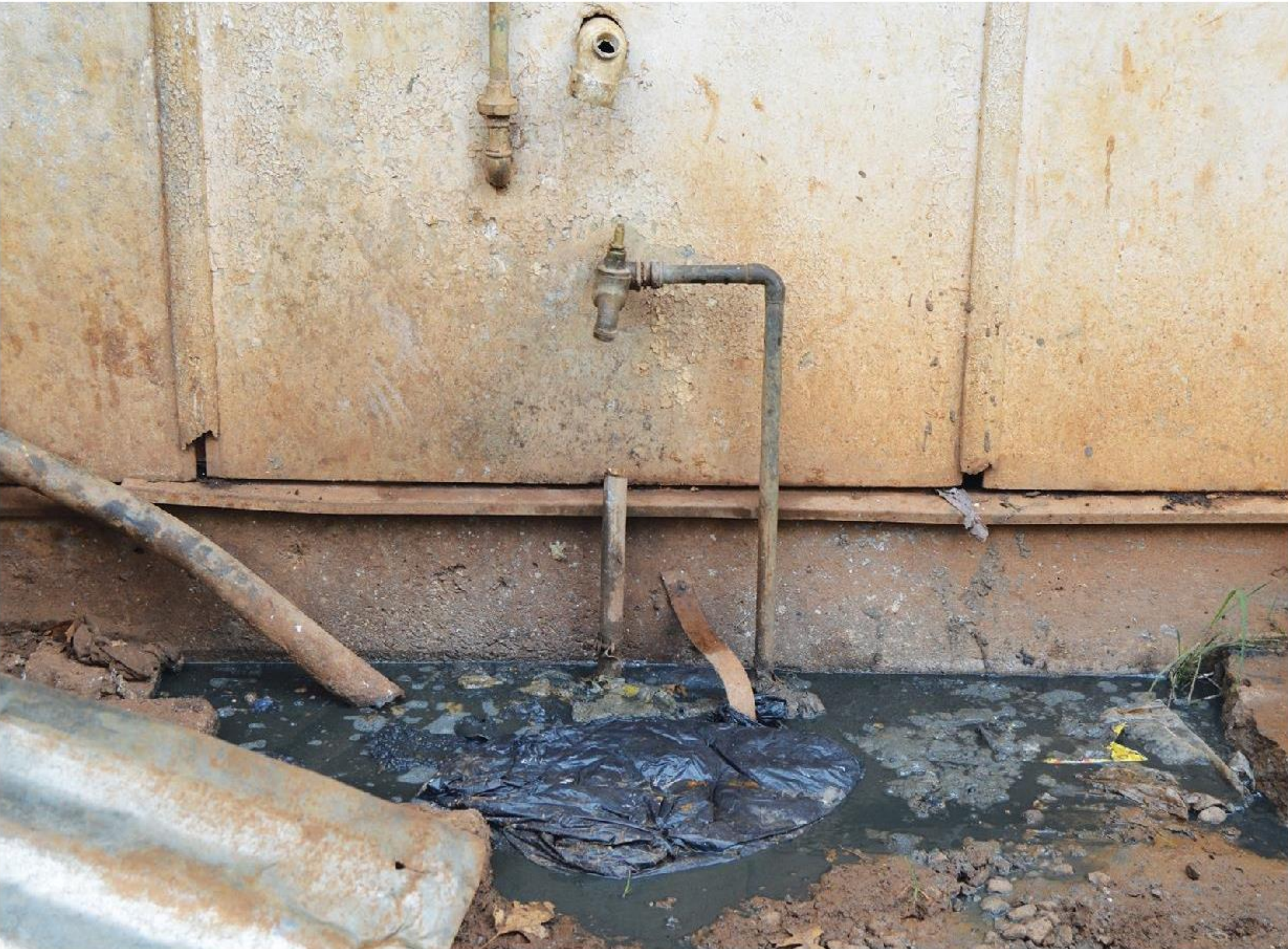
Rising sewage in a drain outside a home, after the occupant has flushed.
