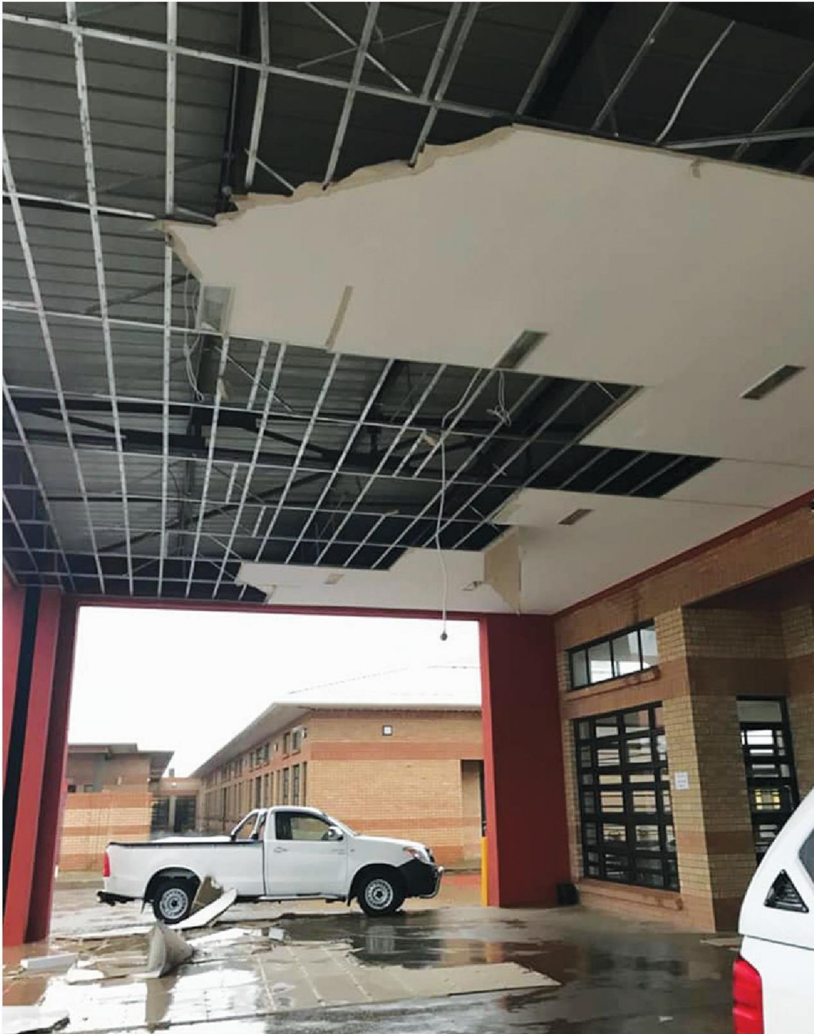
DAMAGE ASSESSMENT: The ceiling at Albert Nzula Hospital’s entrance collapsed after heavy winds and rain in the area.
