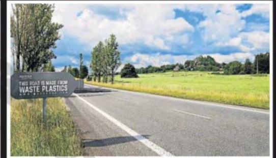
PLASTIC ROAD: Plastic is collected from rubbish dumps, packaged into bales and then melted down with bitumen to make a road
