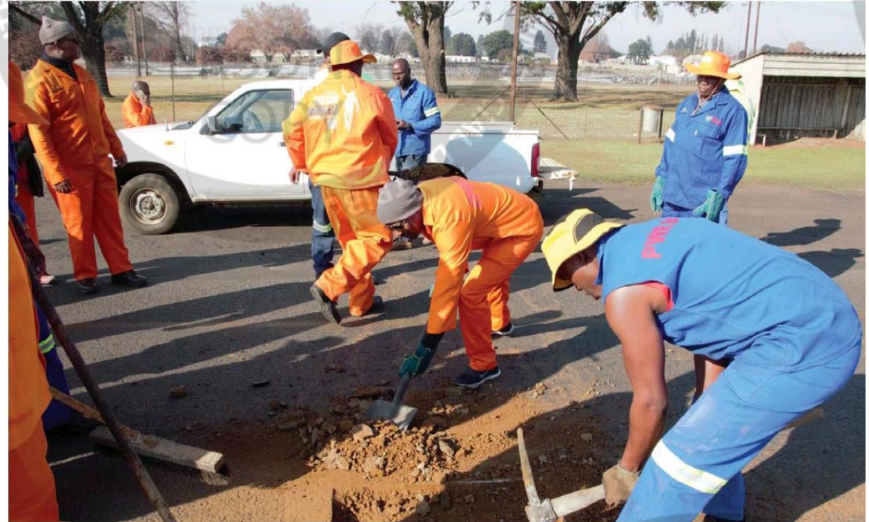
MAKING ROADS SAFER: Public work, roads and transport department workers repairing potholes on the D1398 road near Middelburg.
