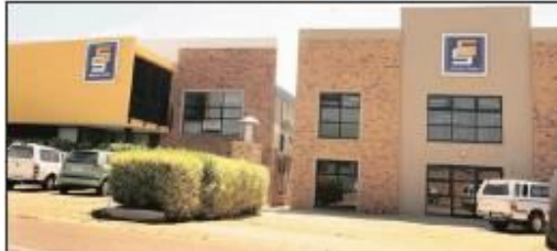
Stefanutti Stocks head offices in Kempton Park, Ekurhuleni. Stefanutti Stocks has identified two emerging companies with which to partner.
