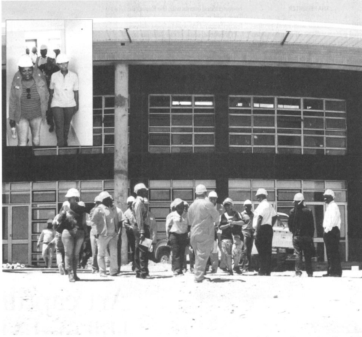
WORK IN PROGRESS: Public works MEC Sisi Mabe and officials inspect the work done on the construction of the Trompsburg District Hospital, giving it the thumbs up.
