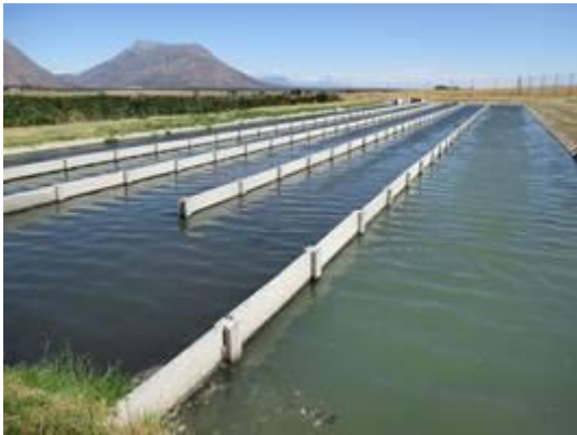
A well-maintained wastewater facility
