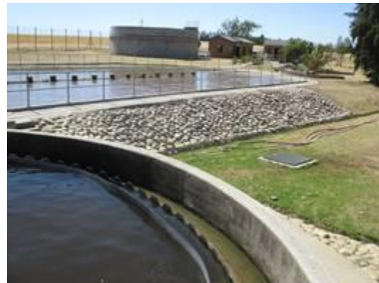
A well-maintained and safe terrain
